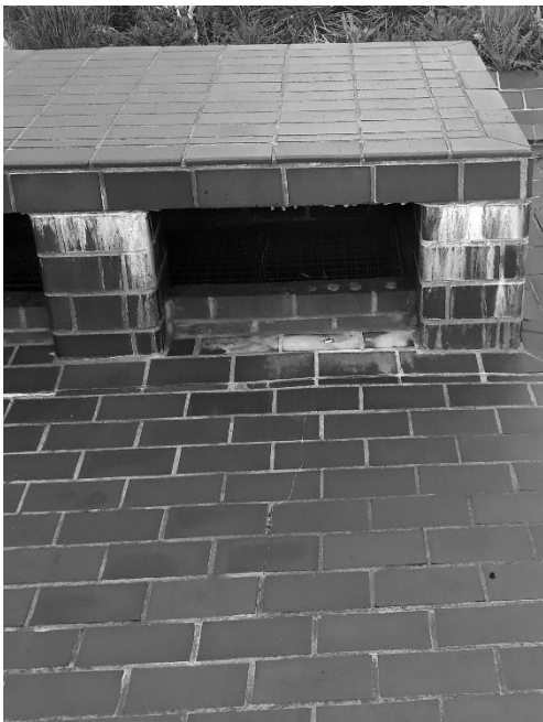
Calcination on a bench on new Beech Gardens Highwalk
