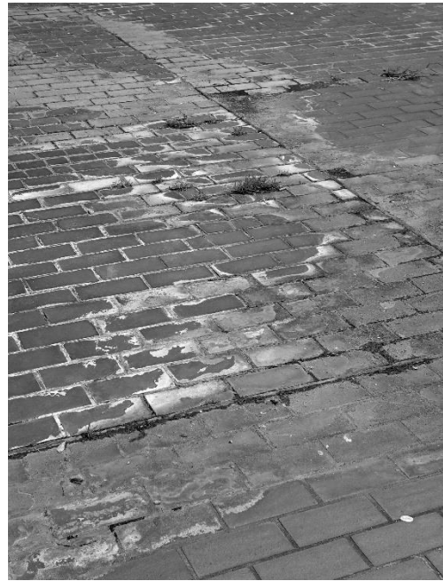
Paving on the Sculpture Court
